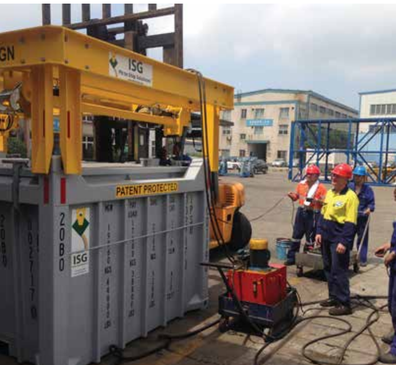
Kevin McCaffrey trialling the hydraulic lid lifter onsite in China
